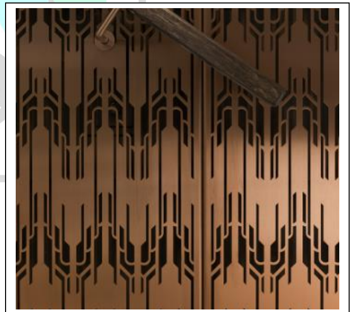
Full height decorative stair balustrading bronze
